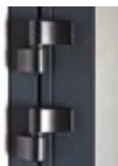
Paumelles et joint anti-pince doigts
